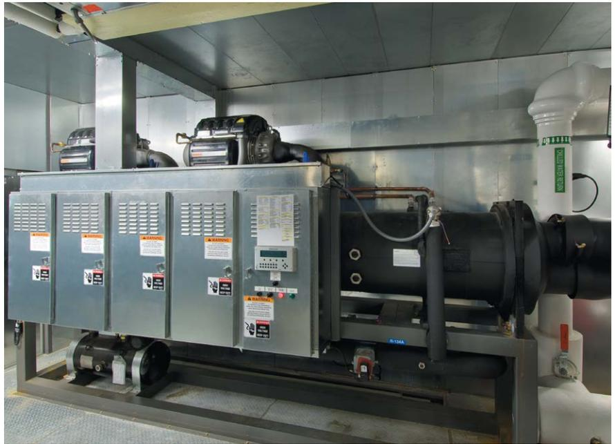
*The innovative, high efficiency packaged chiller plant combines a 500-ton magnetic-bearing centrifugal chiller, evaporative condenser, waterside economizers and controls to provide the highest efficiency and low electrical demand, in addition to quiet operation and reduced maintenance and service.*
