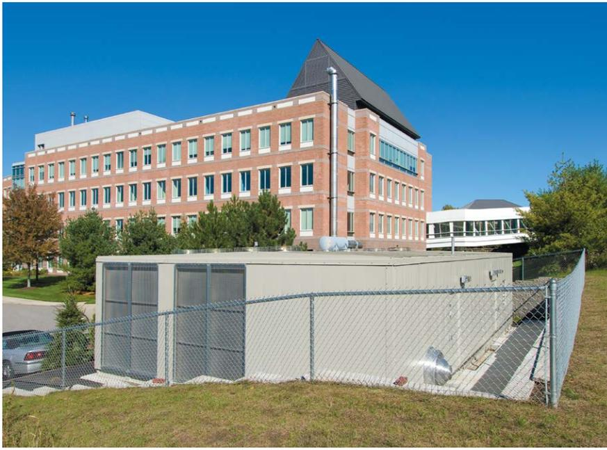
*The Mammoth chiller plant installed at Avid provides a totally self-contained system, precommissioned for plug-and-play operation, sole source responsibility, portability if the facility is vacated, and it meets aesthetic requirements of the building owner.*
